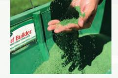
Do not attempt to install the infill material while the synthetic grass or the infill material is wet.
